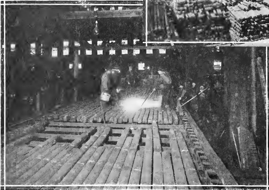
Nicking of Steel Billets by Means of Oxy-Acetylene Torch Preparatory to Breaking by Bulldozer
